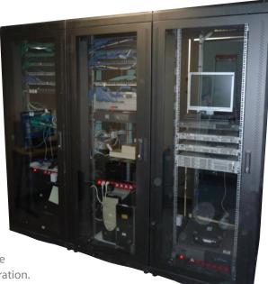
Excel Category 6 cable was chosen to meet all application requirements as it is designed for optimal support of High-Speed data protocols delivering 1 Gbps performance to the workstation. It is also designed to be quick and easy to install. Not only was Category 6 cable installed but also Category 6 patch panels and the associated keystone jacks.
